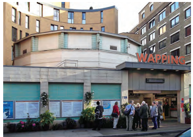
Brunel's shaft at Wapping station
